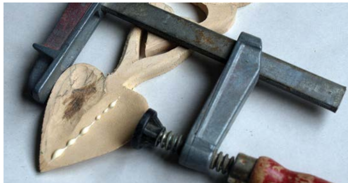
3. If you can clamp the piece without causing further damage, it is generally the best way to achieve a tight, unnoticeable repair. Small fast action clamps are excellent as are the clothes-peg type plastic clamps. Be careful not to damage the wood with excessive clamping pressure.
